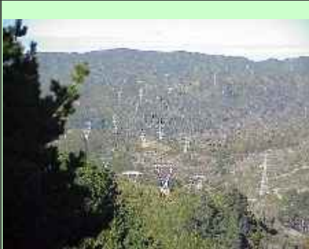
Transmission towers at 41 South, 175 East in New Zealand.
