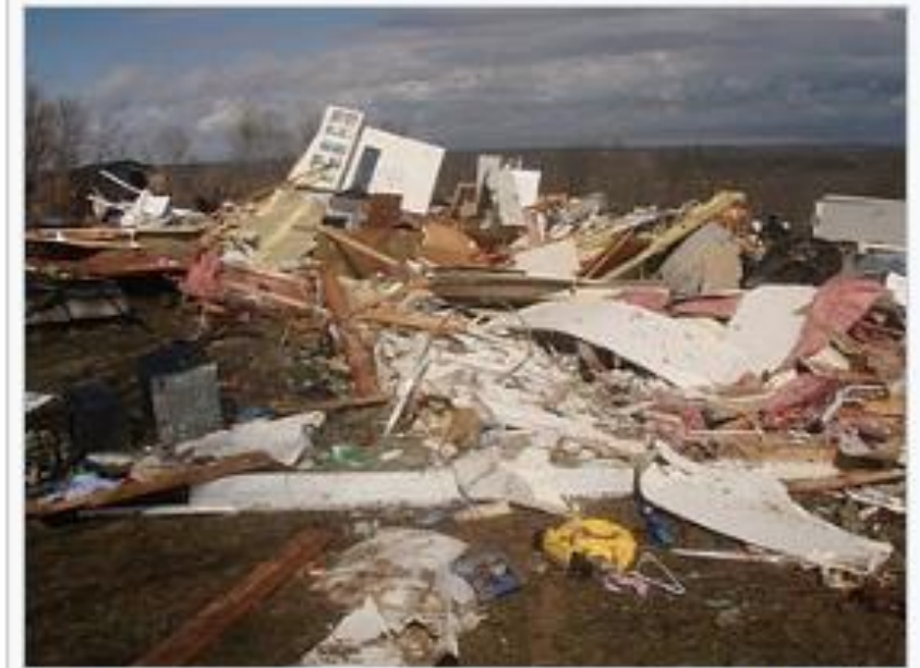
This mobile home was destroyed by a relatively weak EF0 tornado.
